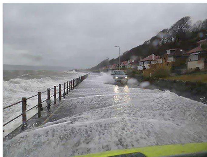
Courtesy TranServ Scotland
